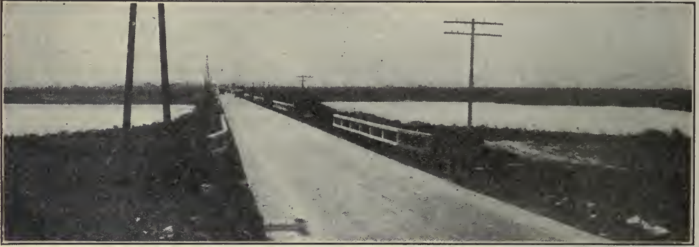
Photo After Carrying Over 4,000,000 Tons Traffic on Los Angeles County Boulevard, equal to 15 years normal use. One of the heaviest trafficked lines in the world.
